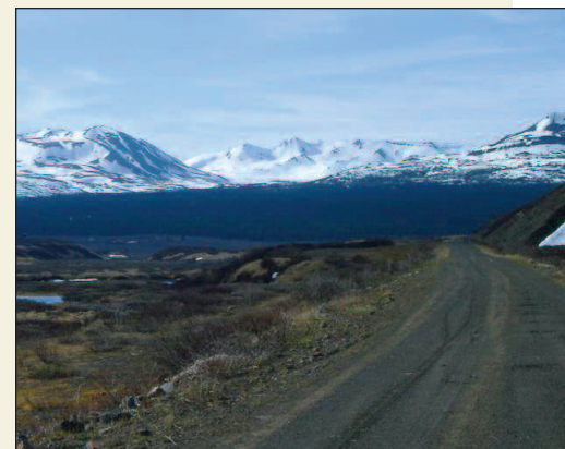
Railway sub-grade links mine site with CN mainline & Ridley Terminals
