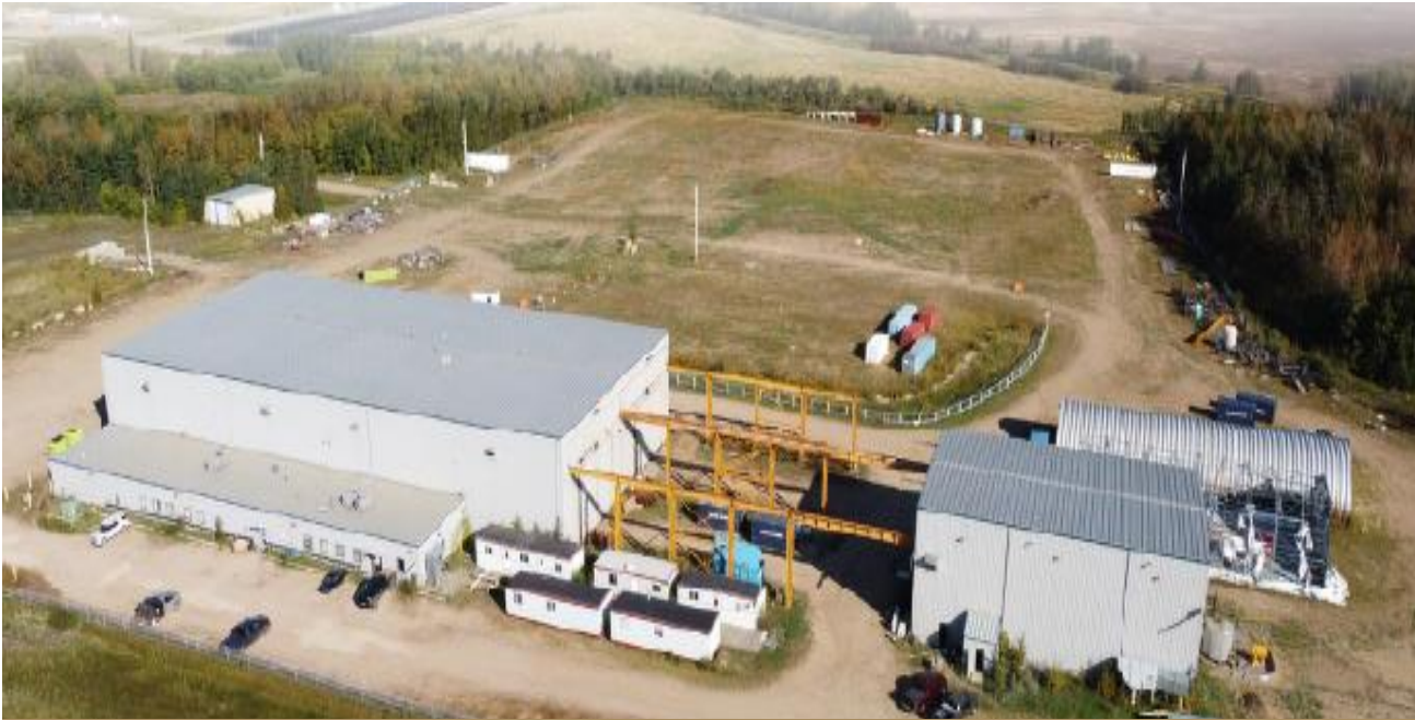
EXISTING PLANT SITE · LAMONT COUNTY, AB
